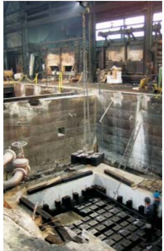
MRM Isolation Elements being lowered into pit using hoist rings.
